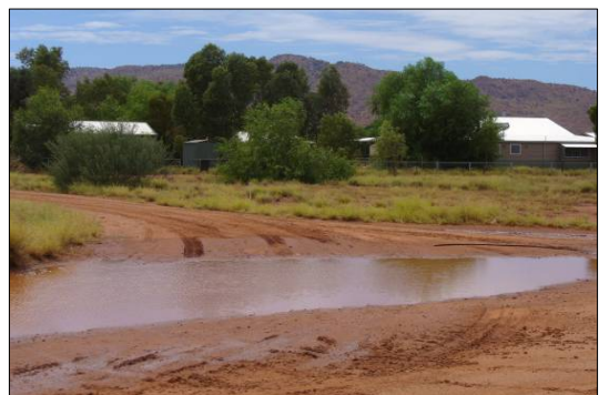
Water pooling after heavy rains
