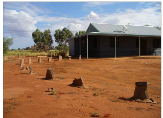
Site for the future Inma area near the office
