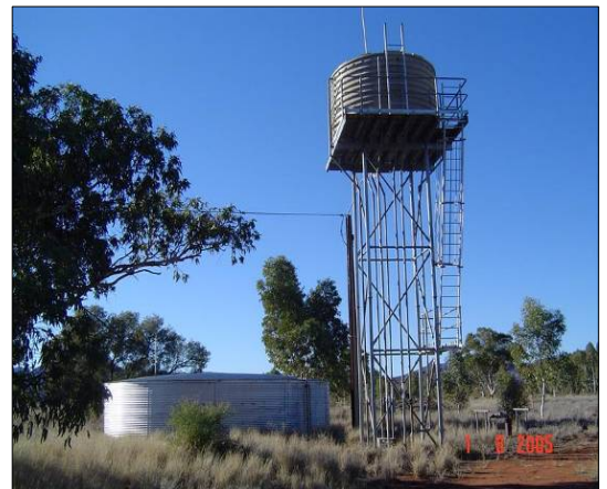
Kanpi water storage tanks
