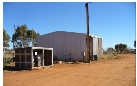
Kanpi workshop and fuel pumps
